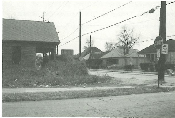
Deterioration in Peopletown.
