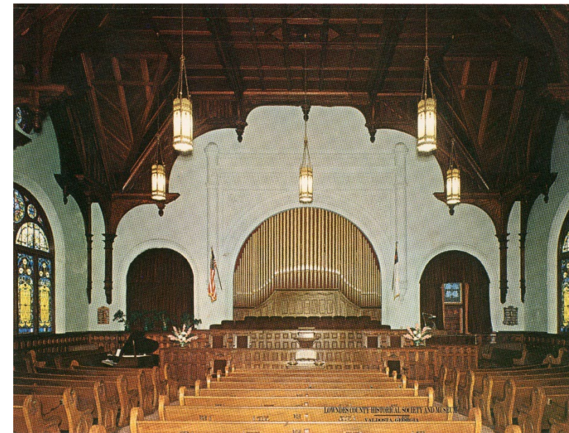
1965 with repainting in progress
