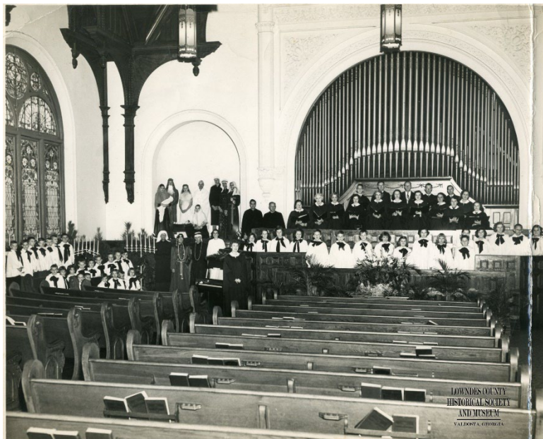
1949 with new luminaires
